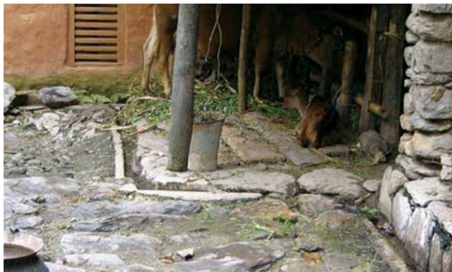
Cattle shed with stone paved floor and urine collection gutter, Okhaldhunga, 2007
