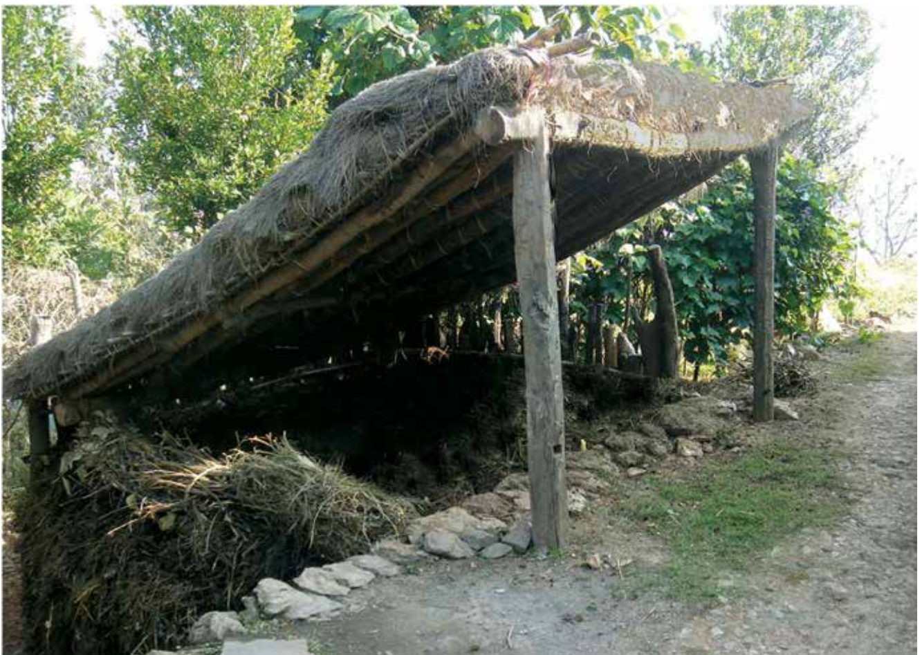
FYM Collection & storage under well thatched roof
