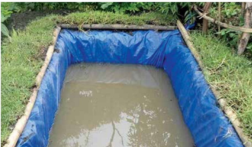
Water collection pond lined with a Silpoulin plastic sheet at a vegetable growing farm, Okhaldhunga, 2013
